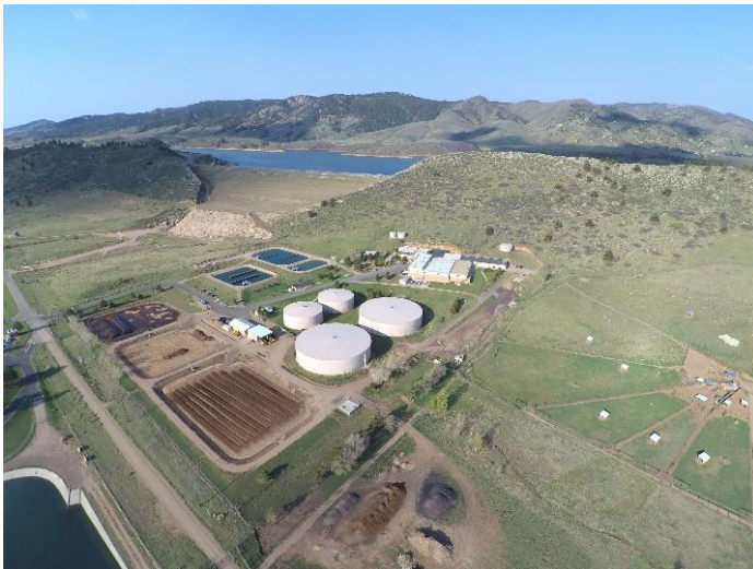
Soldier Canyon Filter Plant
